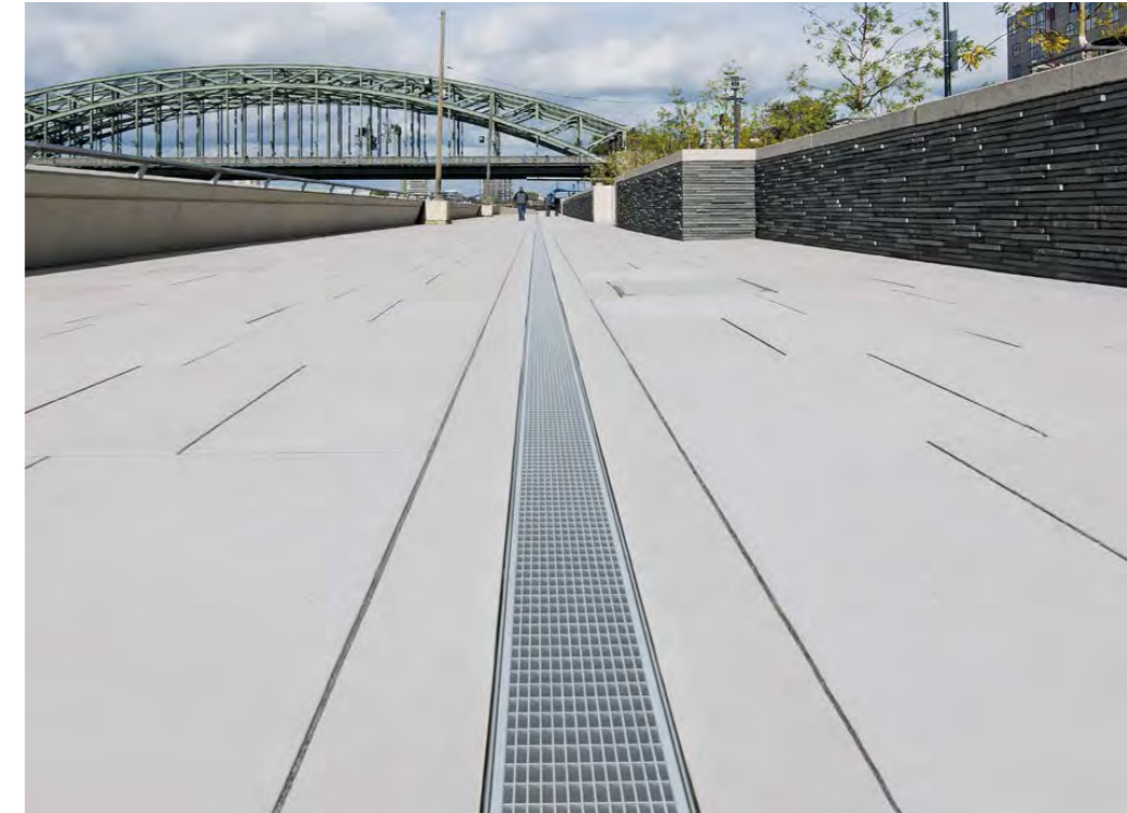
ACO DRAIN® Multiline Seal in am Rheinboulevard in Köln
